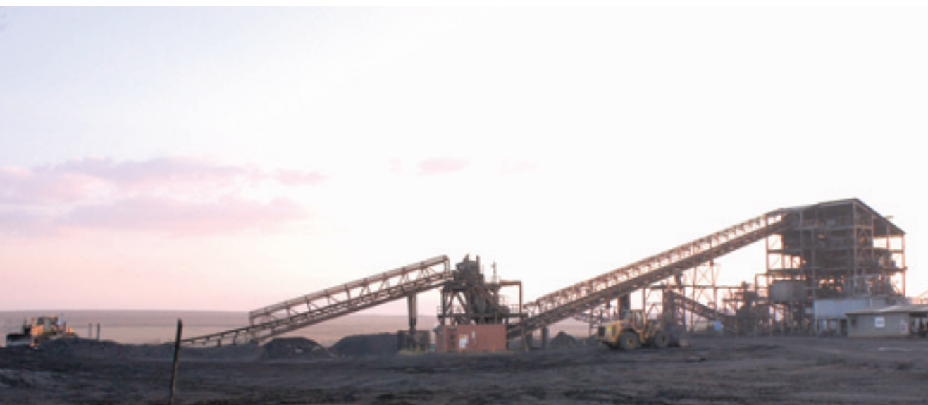
Typical coal crushing and washing plant
